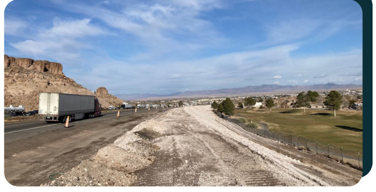
I-40 widening activities near Cerbat Cliffs Golf Course.
