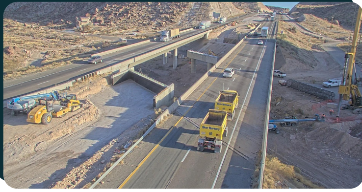
Progress on Clack Canyon Road Bridge widening is continuing.
